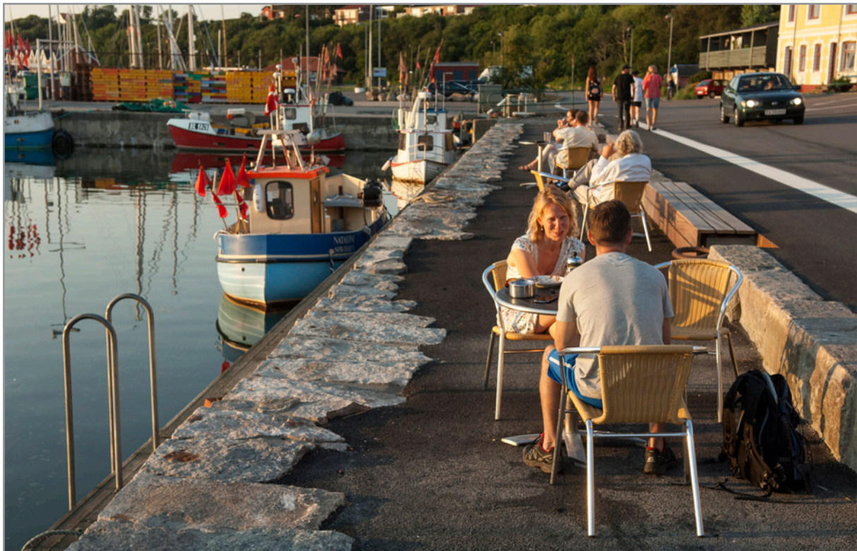
Figure 11: Hasle harbour: the new harbour terraces on the lowered quays at the southern end of the harbour. Photo: Gugga Zachariasdottir.
